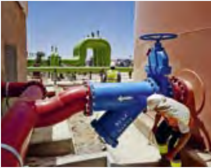
The Noor I Parabolic Trough Power Plant is the first of four ultra-modern solar power plants to go online, in 2015.
